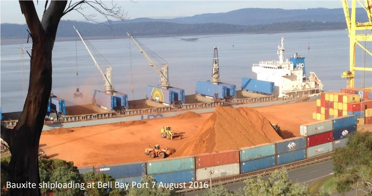
Figure 2: Bell Bay Port of Launceston can handle ships up to 65,000 tonnes. Loading is managed by QUBE Ports at more than 10,000 tonnes per day, achieving 20,000 tonnes per day during a recent loading
